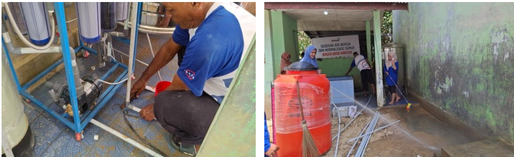
Gambar 2. Pemasangan sistem Smart Water Reservoir
